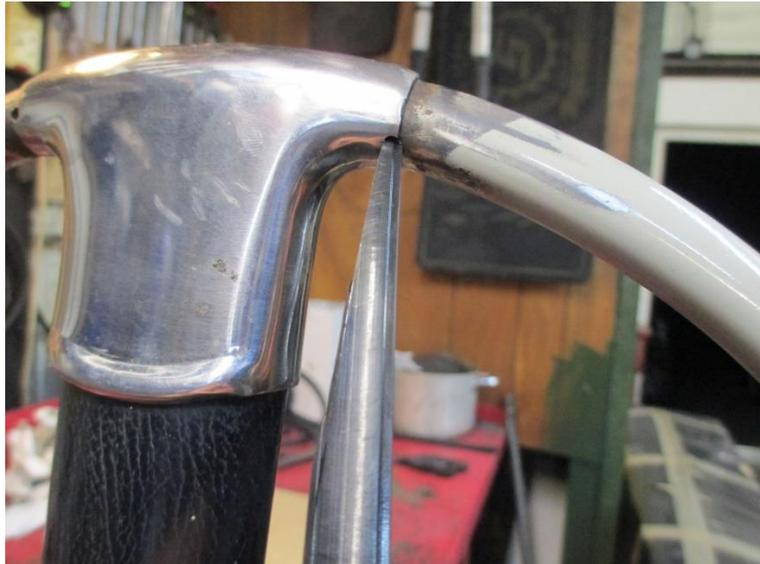
*Picture shows the trimmed end of tape pushed into the hole and ready to begin winding down and away from us.*
